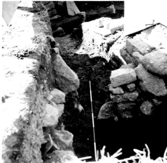
Figure 8 2E-1972 X 2E23J2. Post-excitation shot. 6' scale aligned N-S. Camera facing south.
